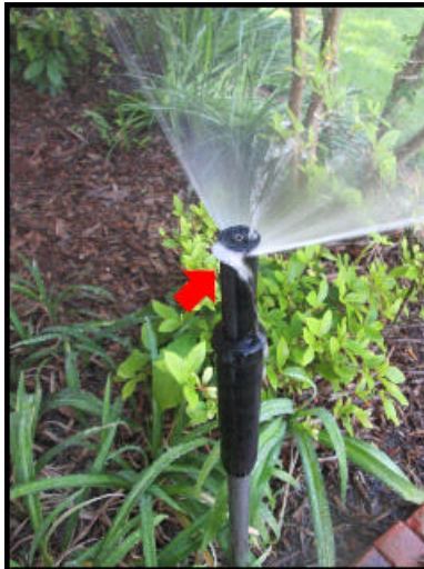
There were 2 damaged heads in this zone.
